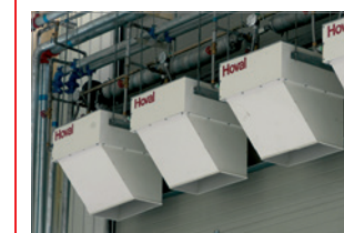
TopVent® curtain prevents energy loss through open doors.
