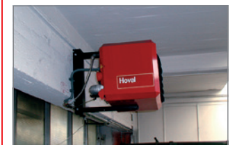
TopVent® GV units are suitable for ceiling or wall installation.
