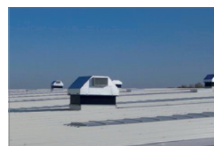
TopVent® commercial units are installed in roofs over high spaces.
