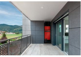
The HomeVent  $^{\otimes}$  comfort ventilation units can be installed flexibly, e.g. also outdoors on the balcony.
