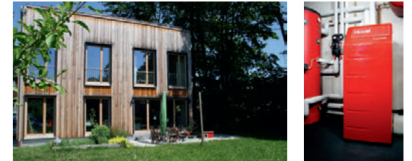
Room heating and water heating using energy from the ambient air.
