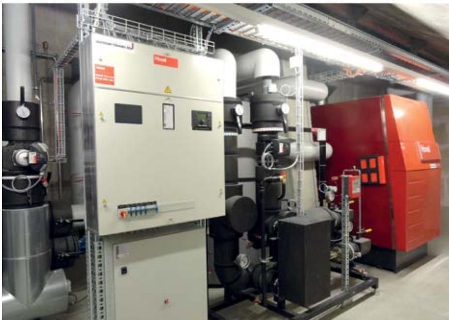
The heating supply for the Velodrome Suisse is taken care of by a Hoval TransTherm 200 transfer station, a custom-produced TransTherm Share heat distributor and a Hoval UltraGas® (500) condensing boiler.
