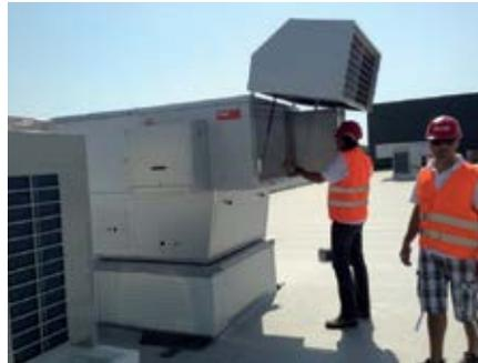
Installation of the Hoval RoofVent® twin pump unit on the roof at MTD Hungária Kft.
